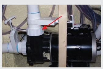
FIGURE 19b : PUMP UNION, LOOSEN UP TO BLEED AIR
