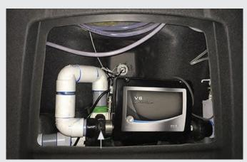
FIGURE 1.9a: HEATER UNION; LOOSEN UP TO BLEED AIR
