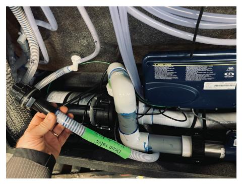
To access it, **remove the panel under the keypad**. The drain hose, identified by a **green sticker**, is located under the spa pack. In some cases, it may be hidden behind the pump.
