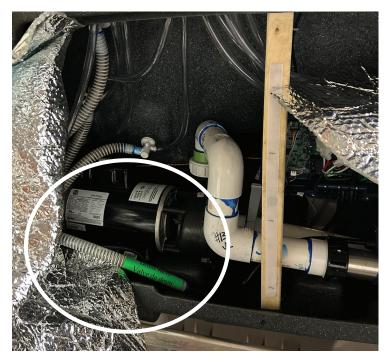
To access it, **remove the panel under the keypad**. The drain hose, identified by a **green sticker**, is located to the right. In some cases, it may be hidden behind spa pack or pump.
