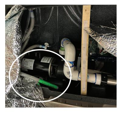
To access it, **remove the panel under the keypad**. The drain hose, identified by a **green sticker**, is located to the right. In some cases, it may be hidden behind spa pack or pump.
