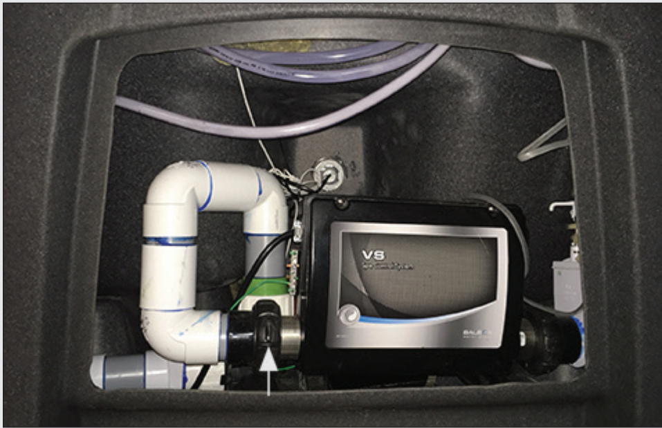
FIGURE 1.9 : HEATER UNION; LOOSEN UP TO BLEED AIR
